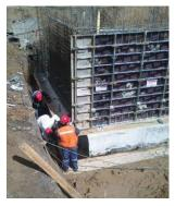
One-component waterproofing coating based on polyurethane and bitumen to seal up difficult to access readings and details. The membrane cures in a continuous and elastic form, as totally adhered layer. This waterproofing layer guarantees total water tightness and withstands building movements.
